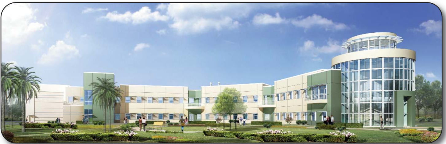
This new construction will add 40,000 sq. ft of laboratory and office space as part of FAU's investment in research at Harbor Branch. (image courtesy of PGAL)
