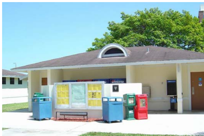
PHOTO 16.20 Trash Receptacles at Modular Building
