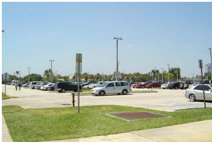
PHOTO 16.2 Parking Lot looking west
