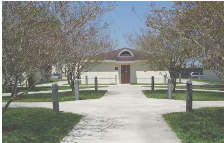
PHOTO 3.7 Courtyard at Modular Classrooms
