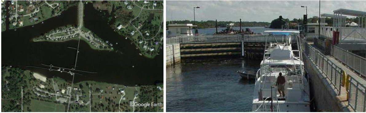
Figure 14. W.P. Franklin Lock and Dam aerial (left) and structure (right) (Google Earth images)
