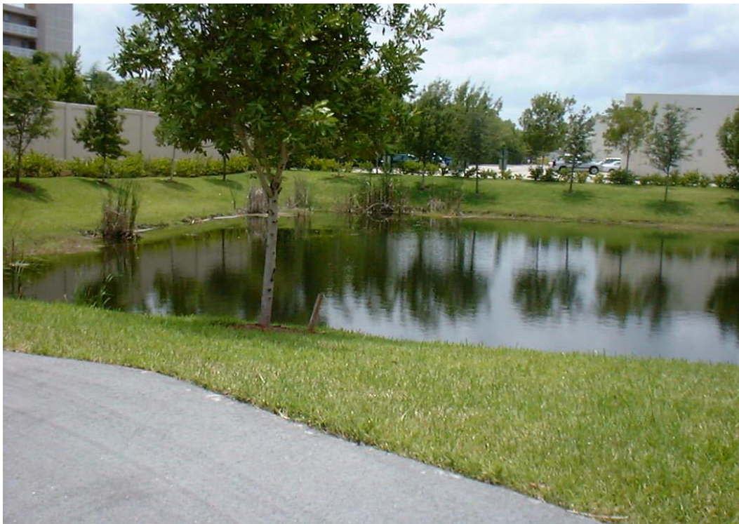
Figure 8. Typical retention pond
