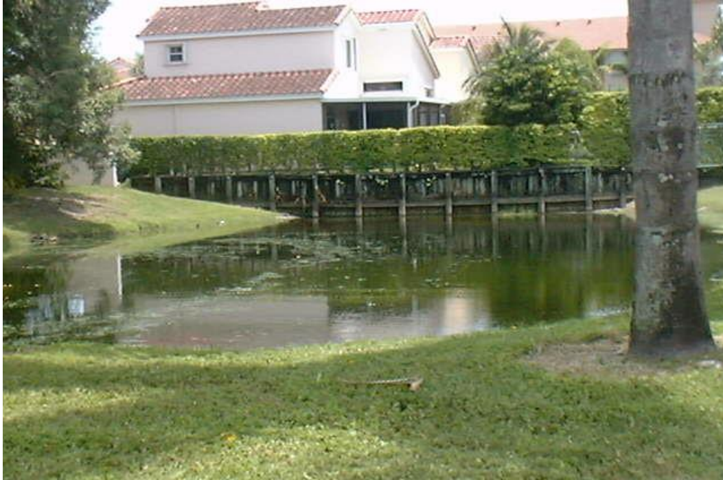
Figure 9. Typical localized canal
