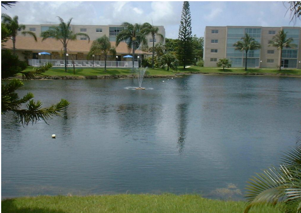
Figure 10. Typical aerated lagoons
